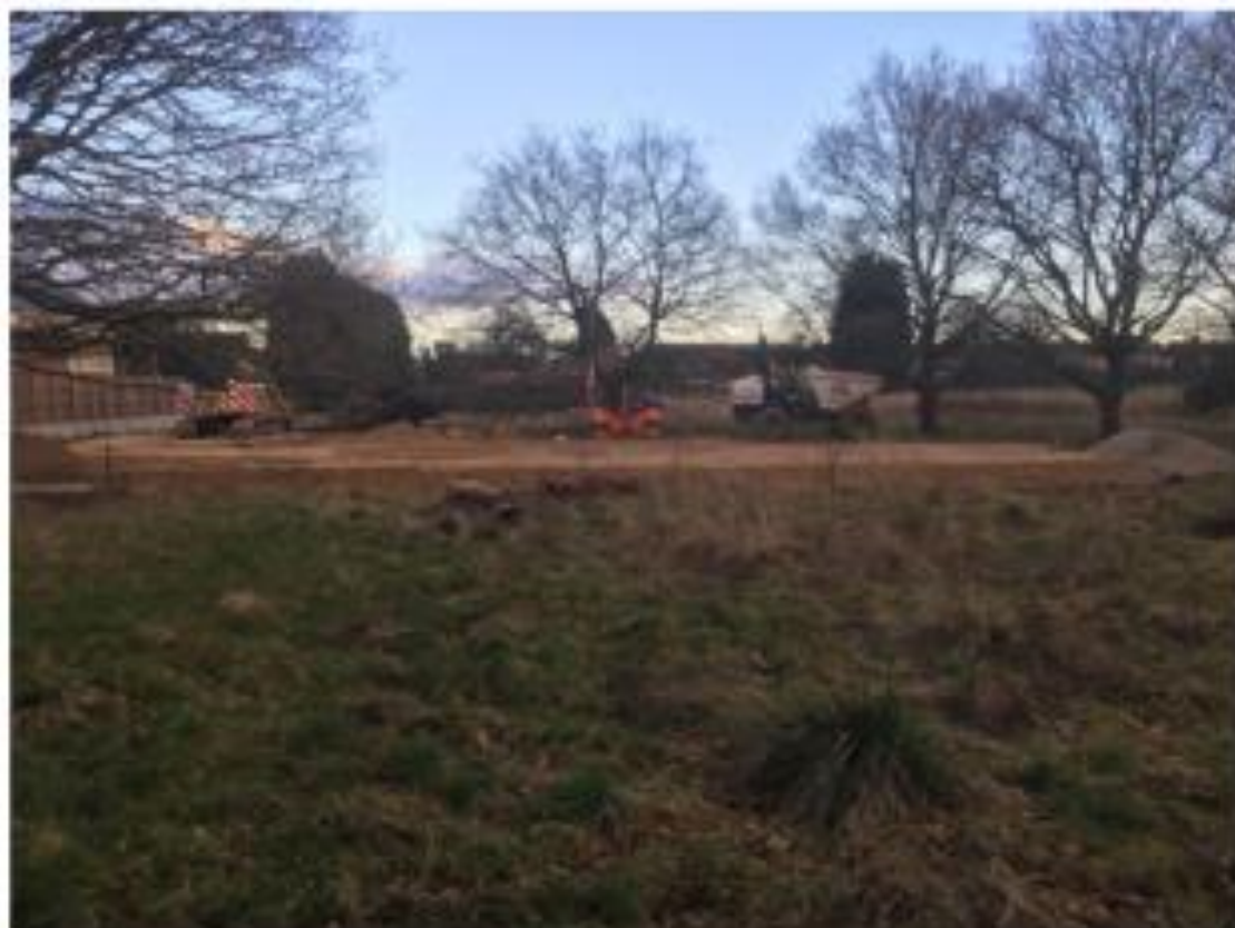
From near Tritton Road , looking across Phase 3 land to the fenced boundary with Phase 2
